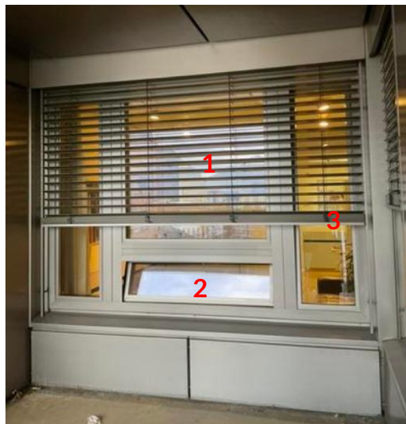
Figure 4. Windows and solar protections
