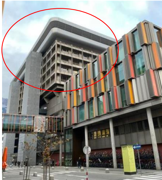
Figure 2. Exterior view of the chosen building
